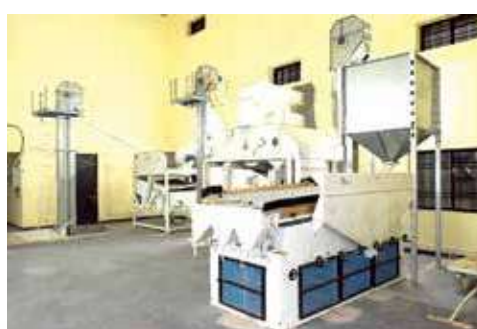
Seed Processing plant
